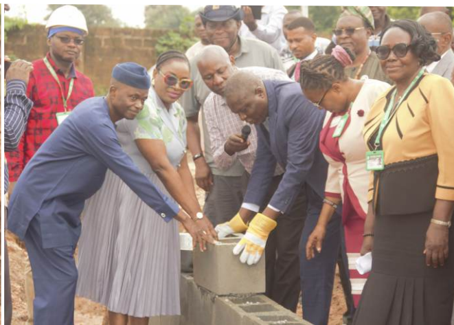
The Medical Director, Federal Medical Centre (FMC), Owo, Dr. Ilyasu Ahmed (in gloves) laying the foundation for the medical students hostel adjacent the FMC, Owo.
