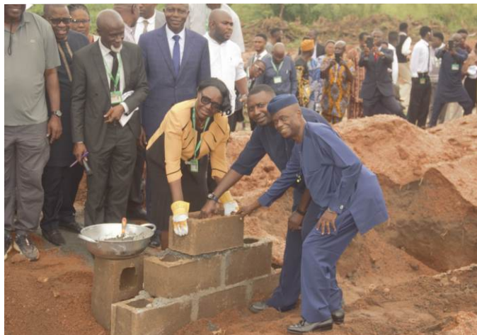
The Vice-Chancellor of Achievers University, Prof. Omolola Irinoye (in gloves) laying the foundation for the academic building within the FMC, Owo.
